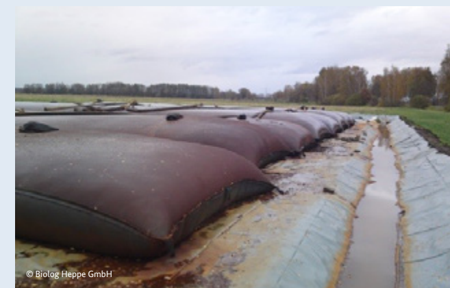
Drainage through Ferrosan geotubes
